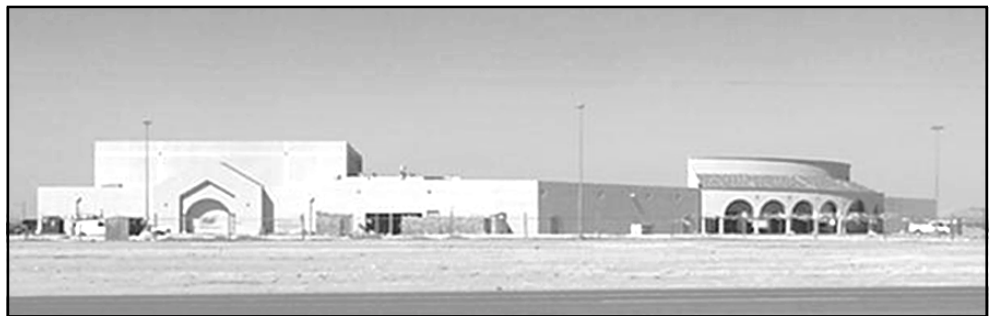
The new Horizon Middle School is scheduled for completion at the end of March 2002. At about 112,000 sq. ft., it will house up to 1,200 seventh, eighth and ninth graders when it opens in August. Clint ISD projects 850 students on the first day of class.
